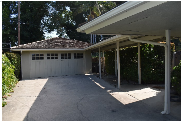
Figure 7. The detached garage, located southeast of the primary residence, contains a pyramidal roof clad in wood shake shingles to match the residence; a portion of the walkway cover is visible to the right, facing north.
