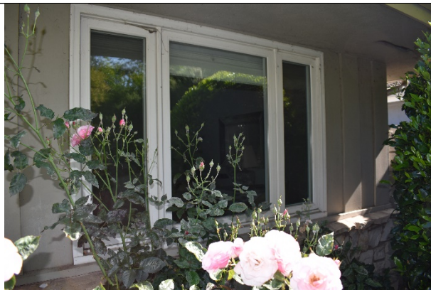
Figure 5. This tripartite wood casement window located on the main (south) is representative of nearly all windows throughout the residence, facing north.
