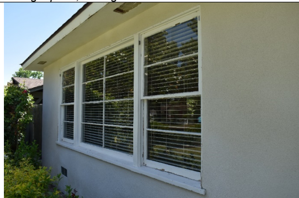
Figure 5. Tripartite focal window on the front (west) façade consists of a fixed central sash and two flanking double-hung sashes, facing north.
