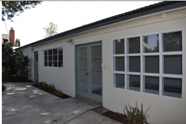
Figure 9. The north façade of the grage features a grid of fixed-pane windows and steel casement windows, in addition to French and standard entry doors, facing southeast.
