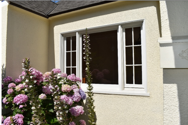
Figure 4. At the front (east) façade, the tripartite focal window consists of a central fixed wood sash flanked by operable multi-pane, wood-sash windows, facing west.
