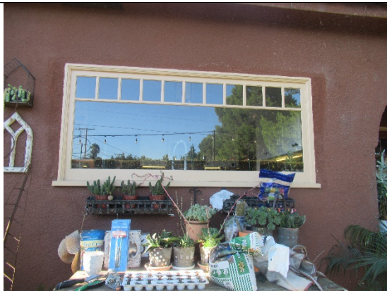
Figure 4. Fixed wood window with upper multi-light transoms, facing south.
