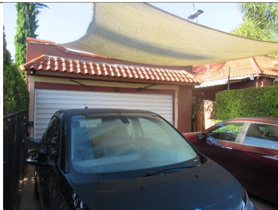
Figure 7. Detached garage with a flat roof with parapet. Clay tile coping wraps around the garage's parapet roofline, with a clay tile roof awning, facing south.
