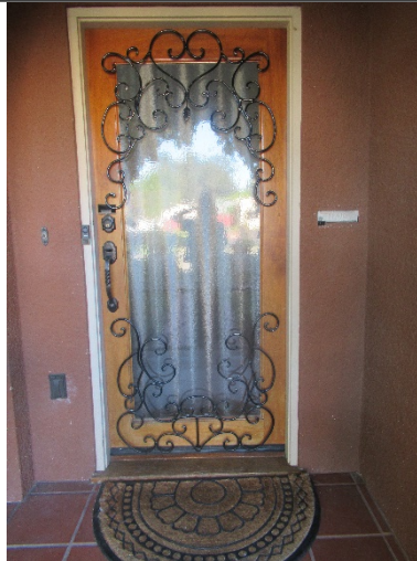
Figure 3. Main entrance door that is composed of a single wood frame door with obscure glass, including metal hardware and decorative metal ornamentation fixed to the door's exterior, facing east.
