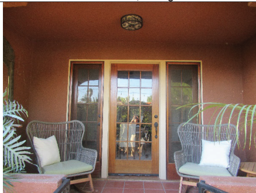
Figure 5. Tripartite wood-frame multi-light side door with a central door flanked by narrower doors, facing south.
