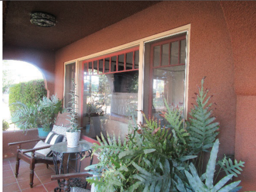
Figure 2. Original tripartite window that has two casement windows with a centered fixed window and upper multi-light transoms at all three window segments, facing northeast.
