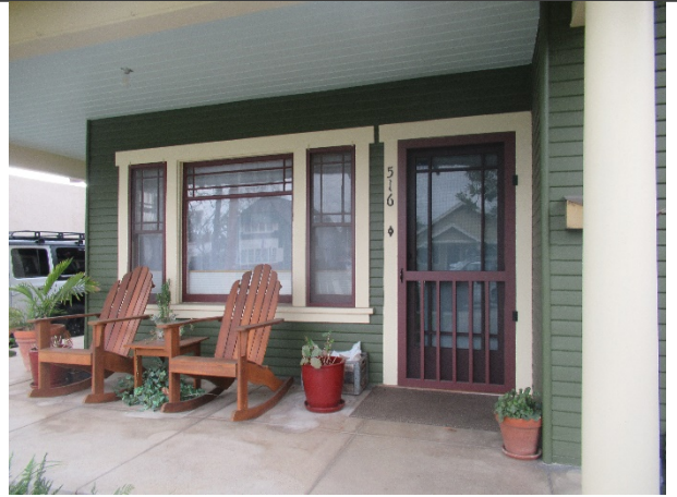
Figure 3. The primary entrance is situated within the covered porch at the primary (north) façade and is composed of a single glazed door with divided lights.
