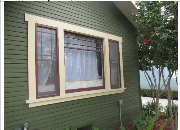
Figure 4. A large tripartite wood-frame windows, comprised of a central fixed window between two narrow double-hung windows with divided lights, adjacent to the main entrance.
