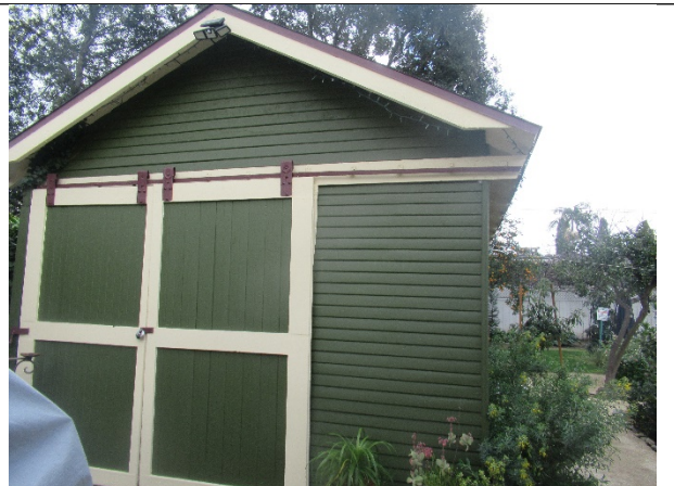
Figure 7. The front-gabled garage has an off-centered vehicular double-door that slides open.
