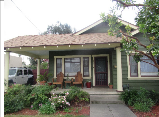
Figure 2. At the primary (north) façade, the covered porch wraps around the building's northeast corner and is supported by three porch columns
