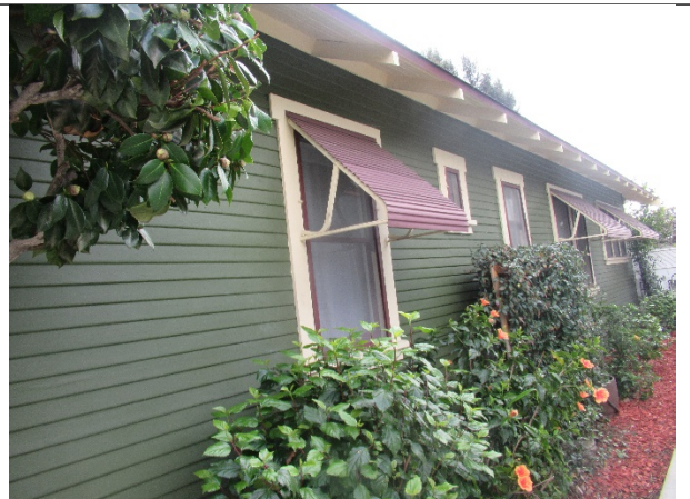
Figure 5. Fenestration on the side (west) façade consists of several double-hung wood windows of various size, along with a small casement window.
