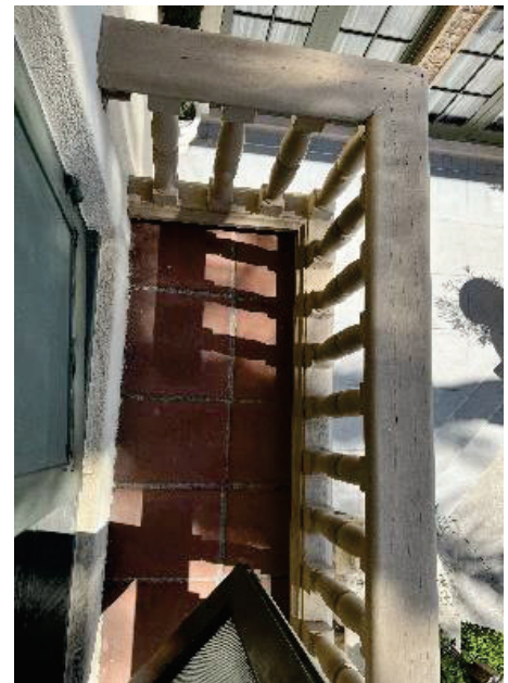
Image 17: The deck's masonry paving appears to be in good condition and currently directs rainwater away for the building.
