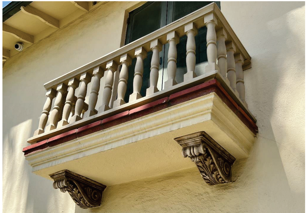
Image 15: The small balconette located on the eastern façade features scroll brackets and a turned wooden balustrade.
