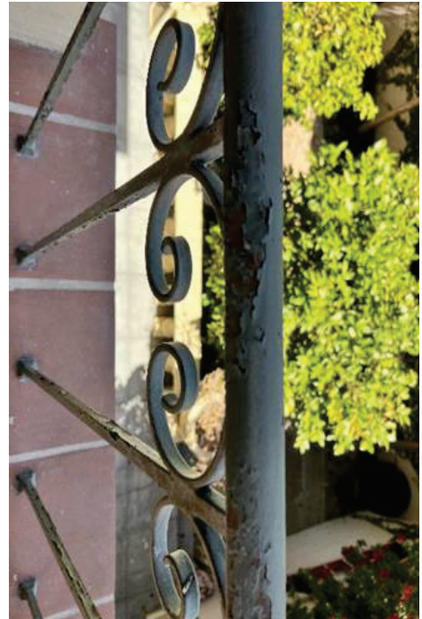
Image 12: Failure of the existing paint coating was also observed. Such loss of the protective coating allows for oxidation of the metal.
