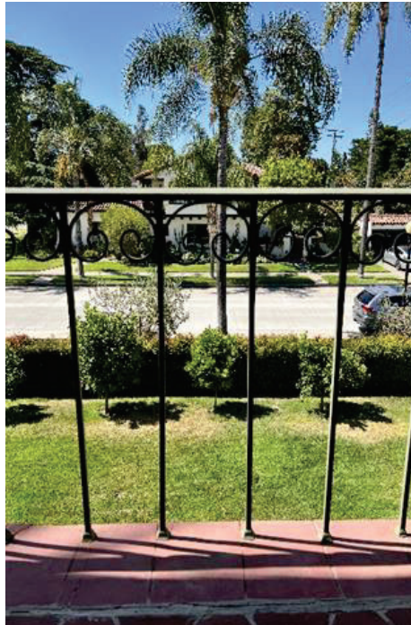
Image 11: The decorative wrought iron rail does not conform to today's safety regulations, creating a potential safety hazard.
