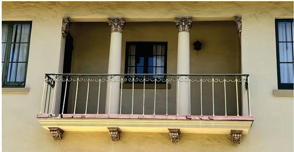
Image 07: South Loggia: The most prominent of the home's second floor balconies includes decorative classical detailing and iron railing. Material losses to the coping are evident.
