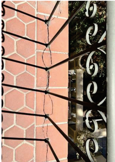
Image 13: Spalling [including losses] was observed where the railing penetrates the concrete coping.
