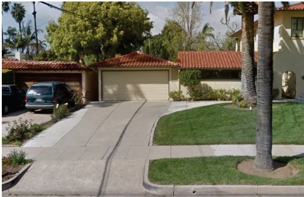
Image 21: 2018 image showing distinctive difference between the old and new concrete visible at both sides of the driveway.
