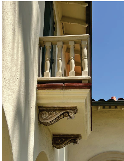
Image 16: Although the railing does not meet current code requirements, the balustrade is in good condition and only requires the removal/replacement of existing paint coatings.
