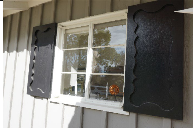
Figure 3. Distinctive board and batten siding, facing northwest.
