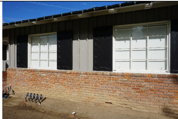
Figure 6. Two identical, steel-frame, multi-lite casement windows, facing north.
