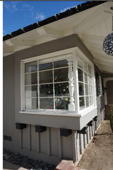
Figure 5. Corner window that projects outward from the façade and wraps around the building's southwest corner, facing northeast.
