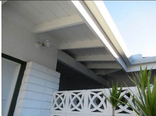
Figure 2. Exposed rafter and continuous fascia detail, facing northeast.
