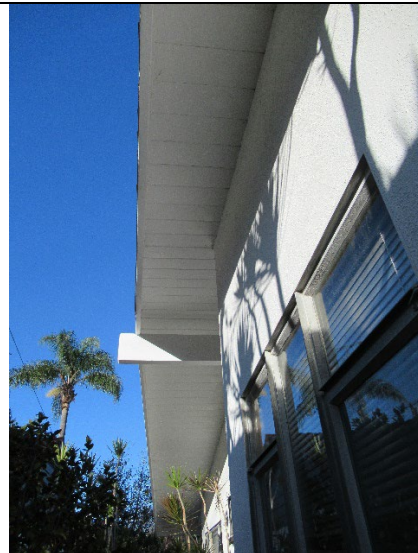
Figure 7. Long beam extending past the gable's end on the south (side) façade, facing west.
