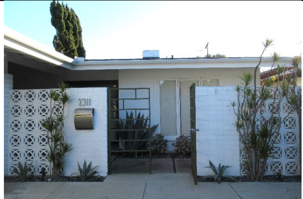
Figure 3. Concrete block brise soleil and whitewashed brick privacy wall, with geometrically patterned wrought iron gate, facing east.
