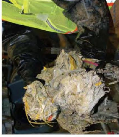
Maintenance crew removing wipes from clogged pumps.
